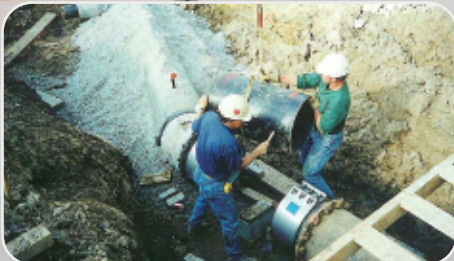
▶ Repair work for pipes replaced underground
