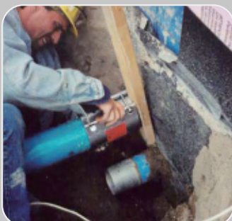
▶ U.S : sewerage repair work
